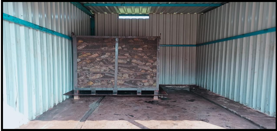
Photo # 14 (C) Used Filters Storage with Secondary Containment
