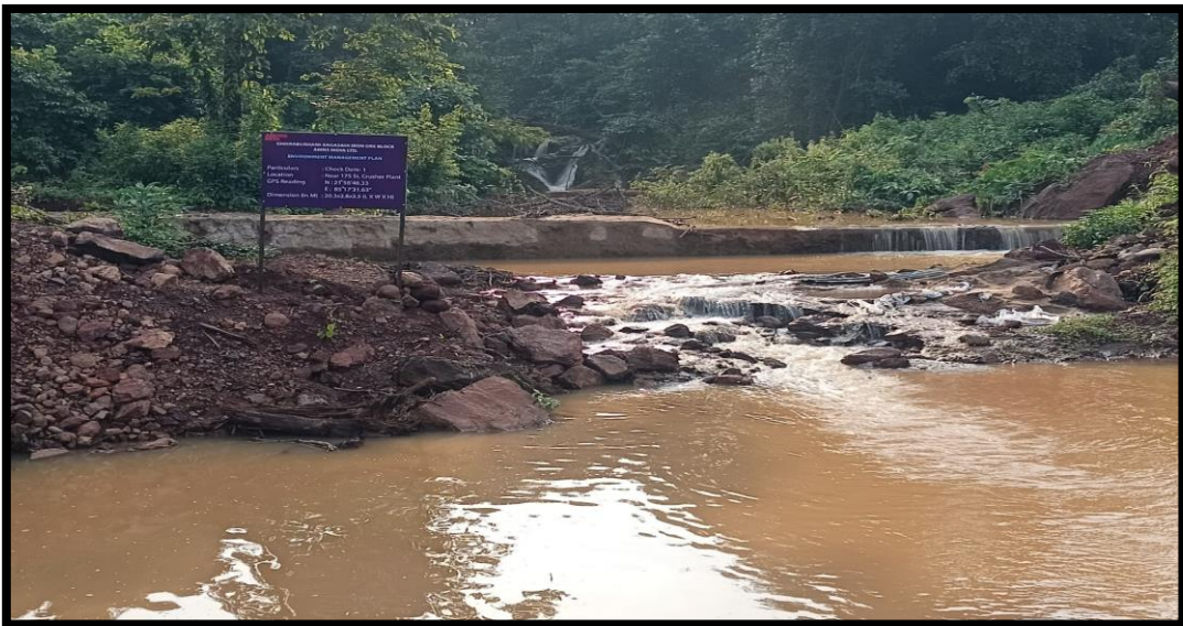
Photo# 2 Construction of Check Dam near 175 TPH Crusher
