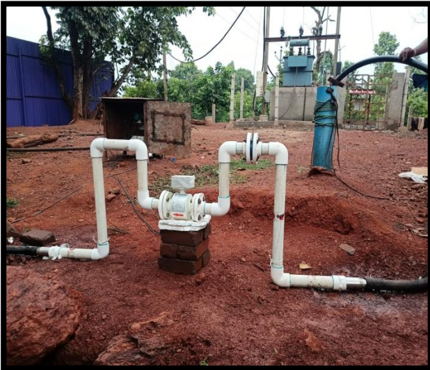
Photo #16(A) (B) &(C) Installation of Piezo Meter & Water Flow Meter with Telemetry System
