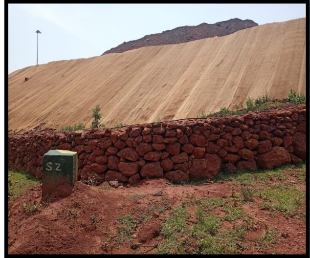
Photo # 12 (A) & (B) Geo textile mat laying on waste dump & fines dump Slop
