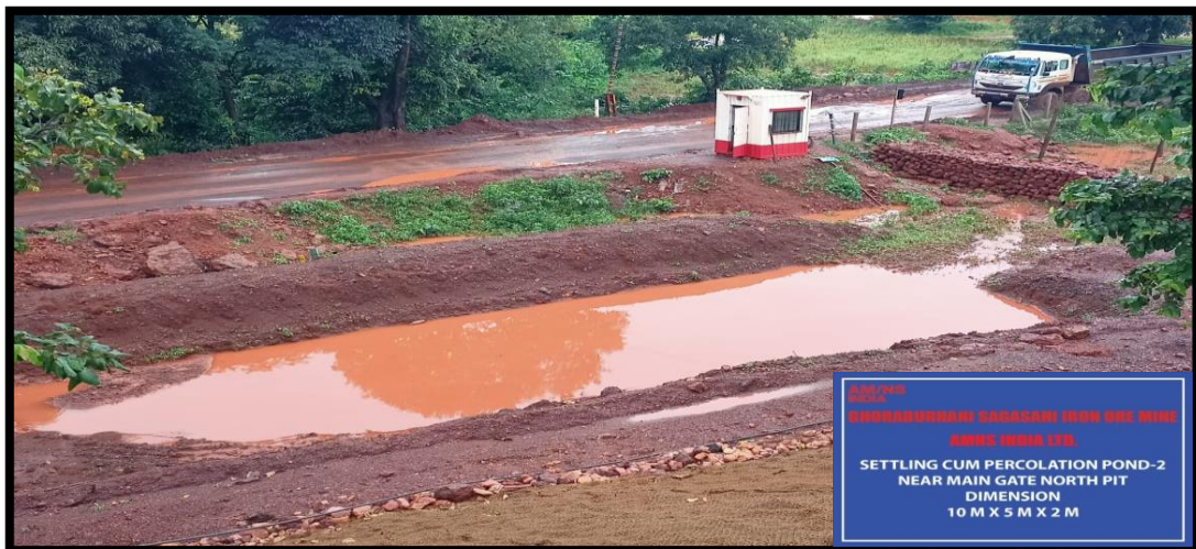
Photo # 9(B) Effluent Treatment Plant at Work Shop
