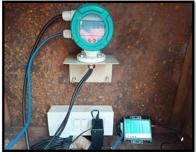
Photo #16(A) (B) &(C) Installation of Piezo Meter & Water Flow Meter with Telemetry System
