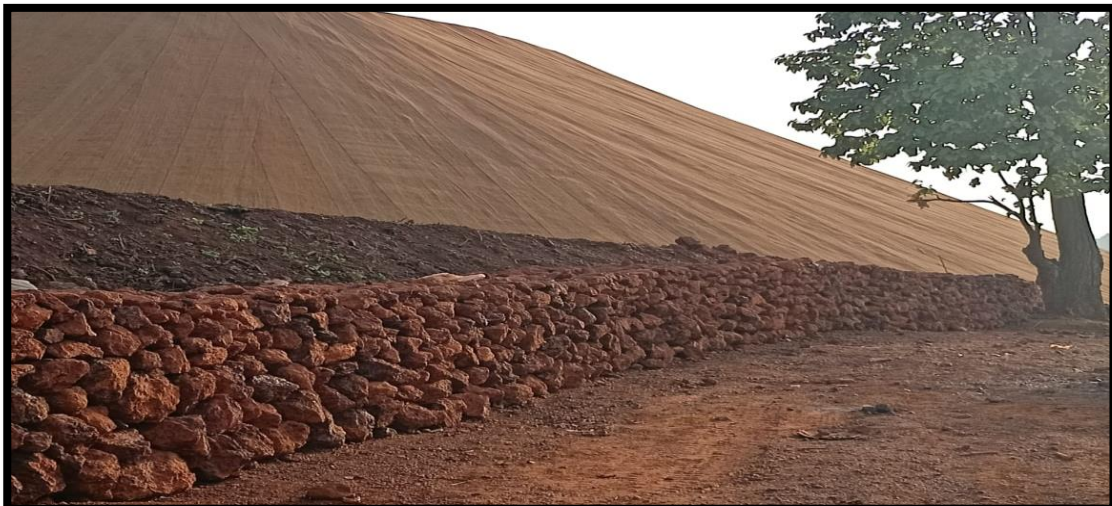
Photo # 10(C) Check Weir provided at sensitive locations
