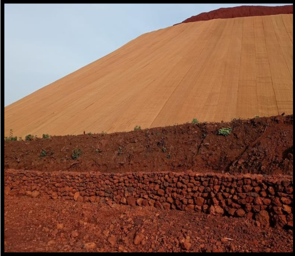
Photo # 12 (A) & (B) Geo textile mat laying on waste dump & fines dump Slop
