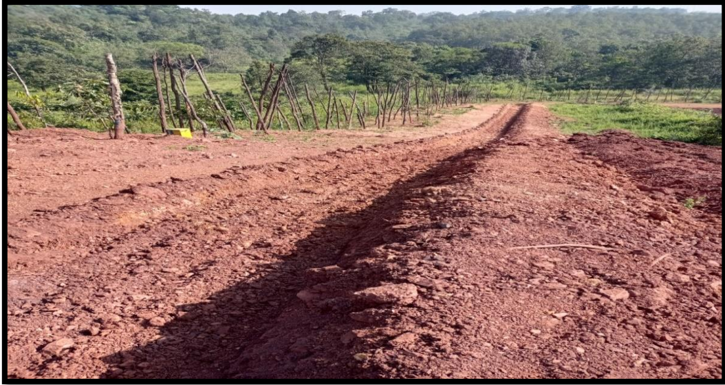
Photo-1 Garland Drain at the toe of OB Dump
