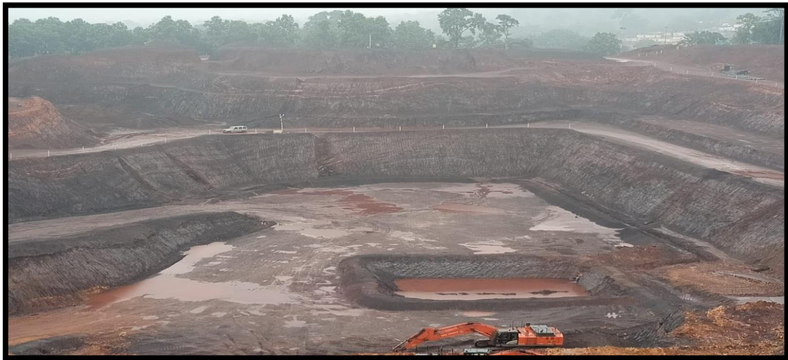
Photo # 13 Pit Sump for collection runoff water
