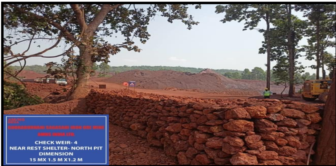
Photo # 10(C) Check Weir provided at sensitive locations
